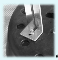
Your pedestal is fastened to the removable lid with aluminum brackets and stainless steel fasteners. The removable lid is attached to the cone with fasteners. accessible from above.
